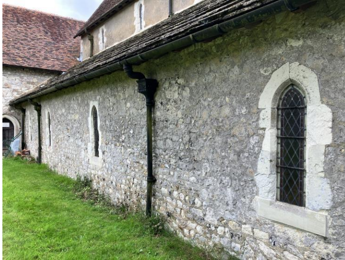
above: The north aisle at low level.
